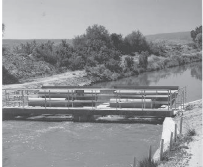
View from downstream.
